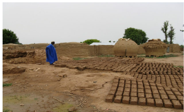
Figure 5. Chief of Dareta halted the brick making process for homes in the village because the bricks made were highly contaminated with lead, contributing to the death of 58 children in 3 months.
