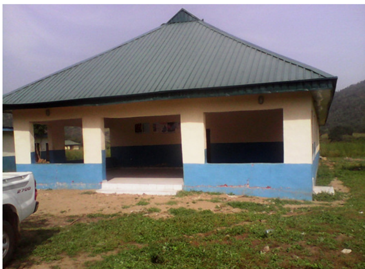
Figure 2: Kujekwa primary health center centre in Abuja, Nigeria - 2014
